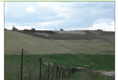
Northeast slope - airspace recovery
